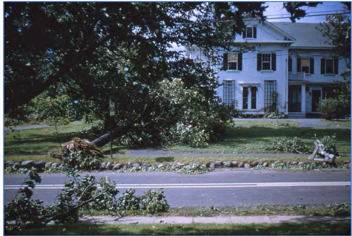
Figure 15. Damage from Hurricane Carol on East Main Street.
